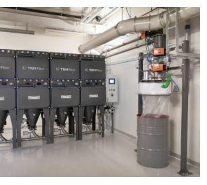
Dedusting filter system type ECR by TRM Filter with central dust collection and continuous liner in pharmaceutical application.
